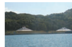
7. Maehata Munitions Depot A munitions depot that was built in 1889 and continued to be expanded until the end of World War II.
