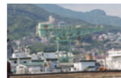
4. Tategami Basin and the Hammerhead Crane A structure consisting of a basin and crane that measures 576 meters wide by 363 meters deep in order to accommodate huge warships. They were completed in 1913.
